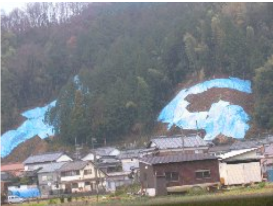
Landslide sites covered by plastic sheeting
